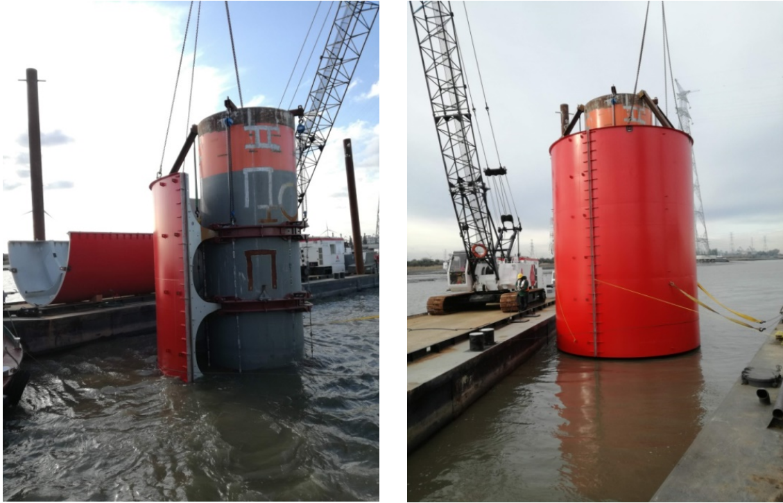
Fig.3. Installation of caisson structure attached to pile
