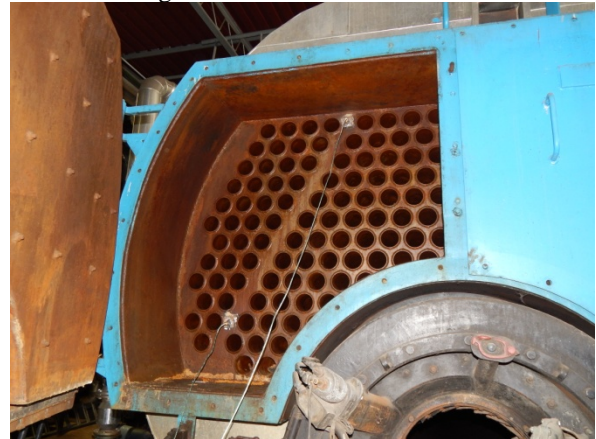
Fig. 1 Installation of temperature probes
